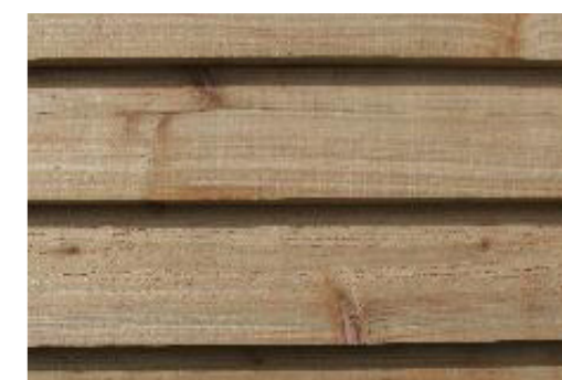
Feather-edged weatherboarding for garage structure
